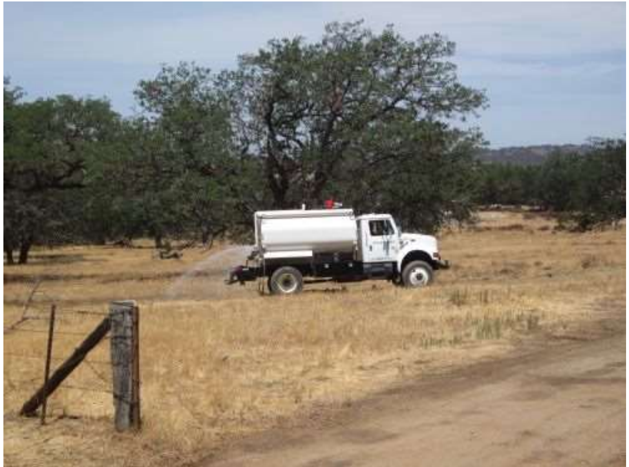
Photo 1: Trucks were observed applying water along project access roads in order to prevent fugitive dust in accordance with APM BIO-1.
