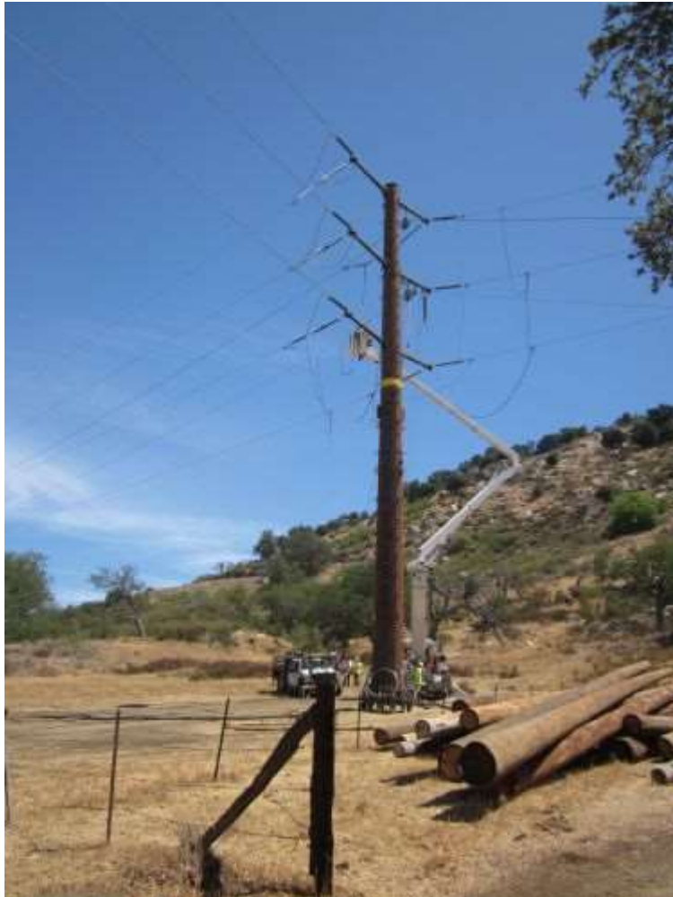
Photo 7: Between Locations 151 and 163, wire pulling for the 69kV line was observed.
