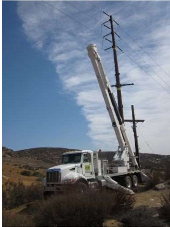
Photo 5: Construction crews were observed preparing to hang davit arms at Location 71.
